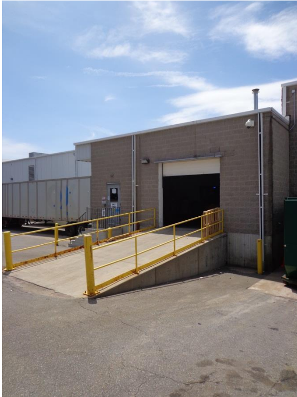
Figure 6. Kraft plant entrance, Wausau, WI
