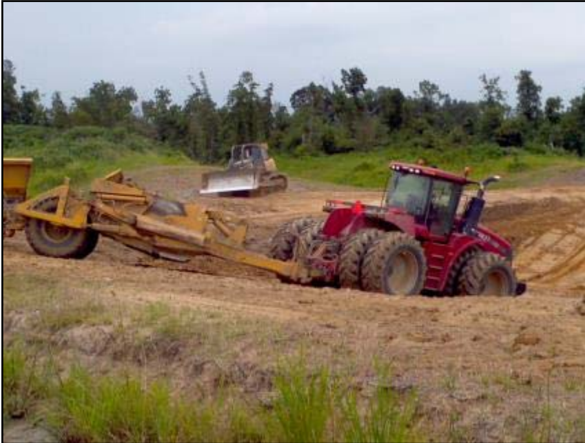
A tractor removes overburden at Old Ed Carbon Recovery Site.
